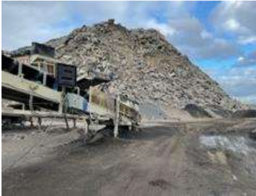
Photo (35): Pave AL Crusher: 1250 Shawson Dr., Mississauga, ON
