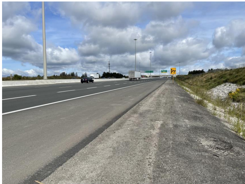
Figure 19. Highway 400- NB – Before King Road Bridge - No Distresses (September 2022)
