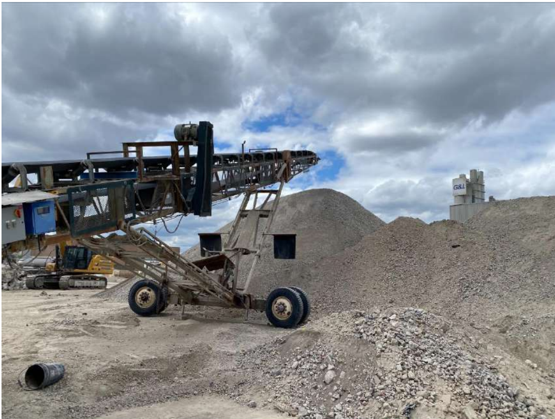
Photo (26): Strada Aggregate Crusher: 120 Wentworth Crt, Brampton, ON – Producing RCA
