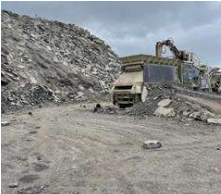
Photo (36): Pave AL Crusher: 1250 Shawson Dr., Mississauga, ON
