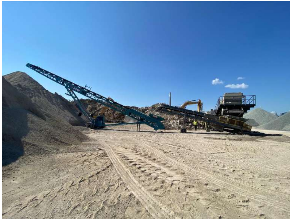
Photo (29): Strada Aggregate Crusher: 10 Leslie St, Toronto, ON– Producing RCA
