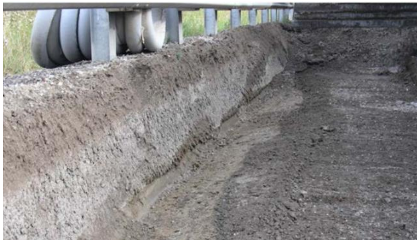
Figure 39. Highway 427 – New Highway Constructed Adjacent to Existing Highway
