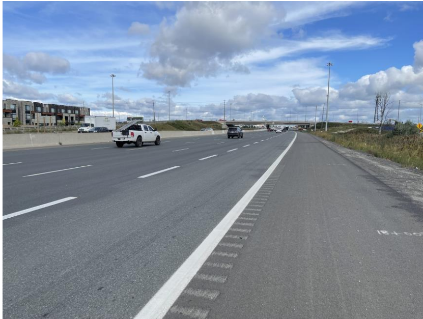
Figure 18. Highway 400- NB – Before Teston Road Bridge- No Distresses (September 2022)
