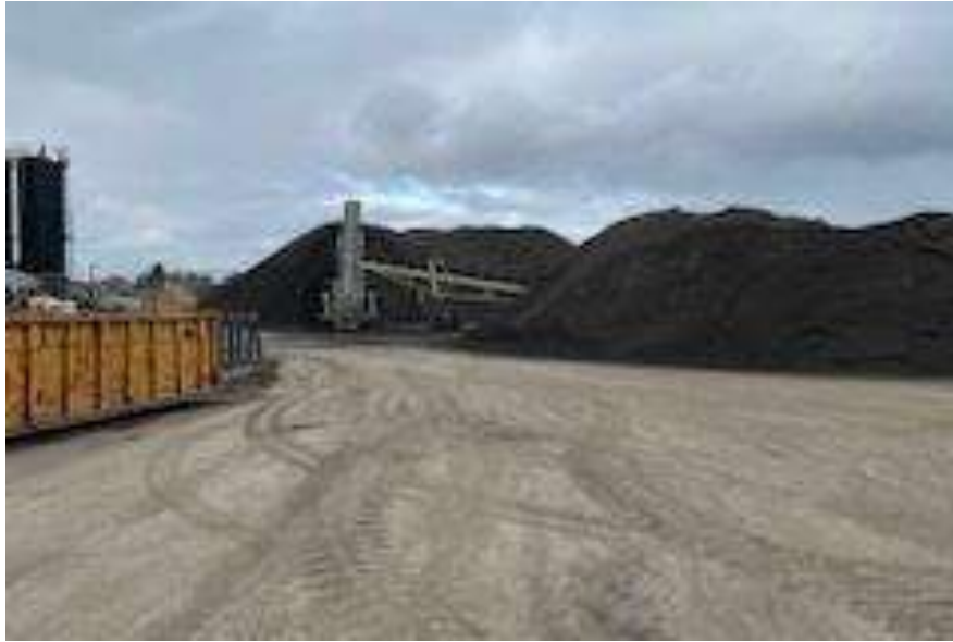
Photo (37): Pave AL Crusher: 1250 Shawson Dr., Mississauga, ON
