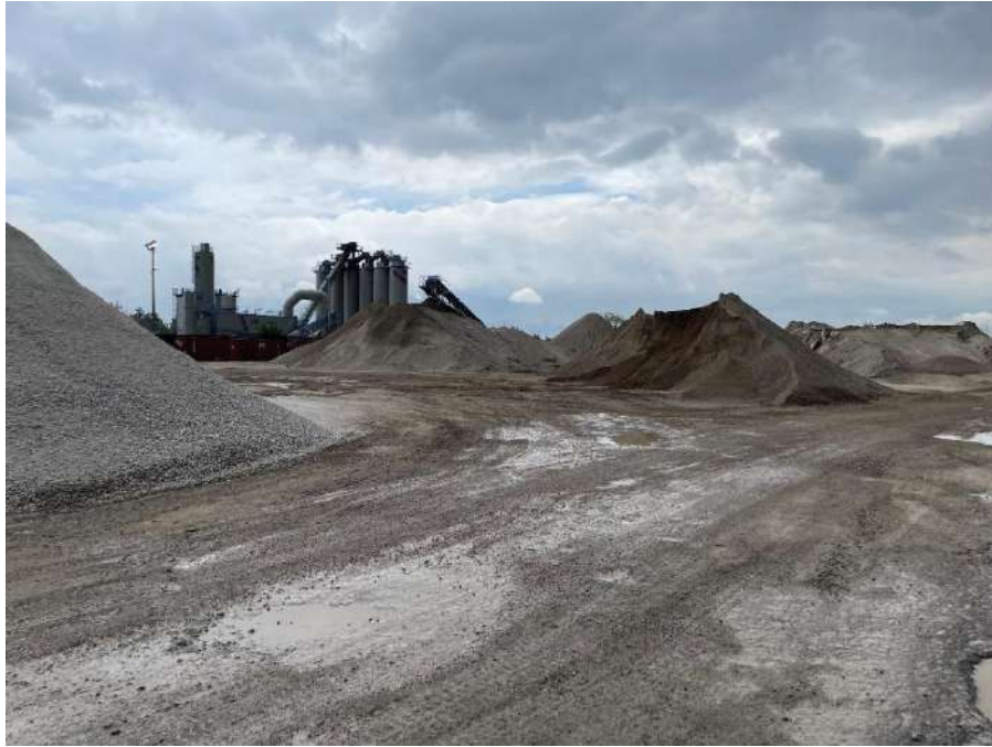
Photo (15): Crupi Crusher at 2777 14th Ave, Markham- Stockpiles of Produced RCA and RAP
