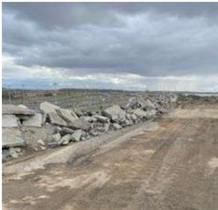
Photo (40): Pave AL Crusher: 1250 Shawson Dr., Mississauga, ON
