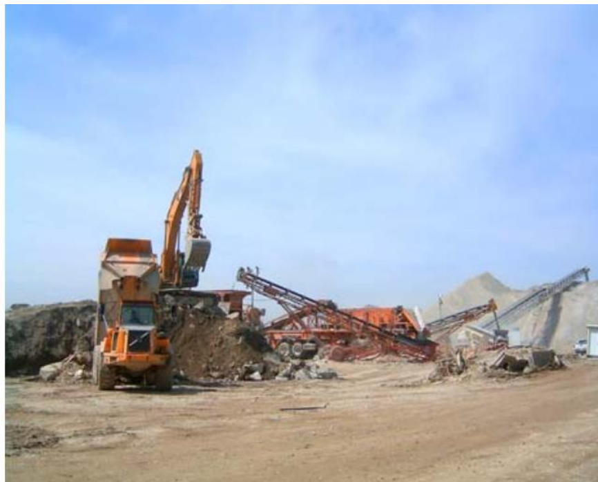
Figure 14. Pearson International Airport – One Site Concrete Crushing Plant and Processed Concrete Backfill (2004)
