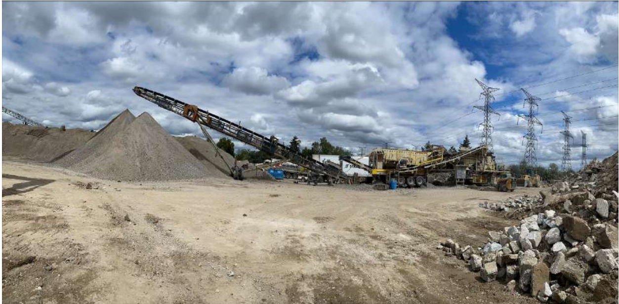
Photo (25): Strada Aggregate Crusher: 120 Wentworth Crt, Brampton, ON – Producing RCA
