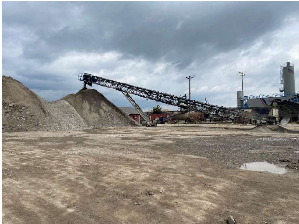
Photo (11): Crupi Crusher at 2777 14th Ave, Markham, ON
