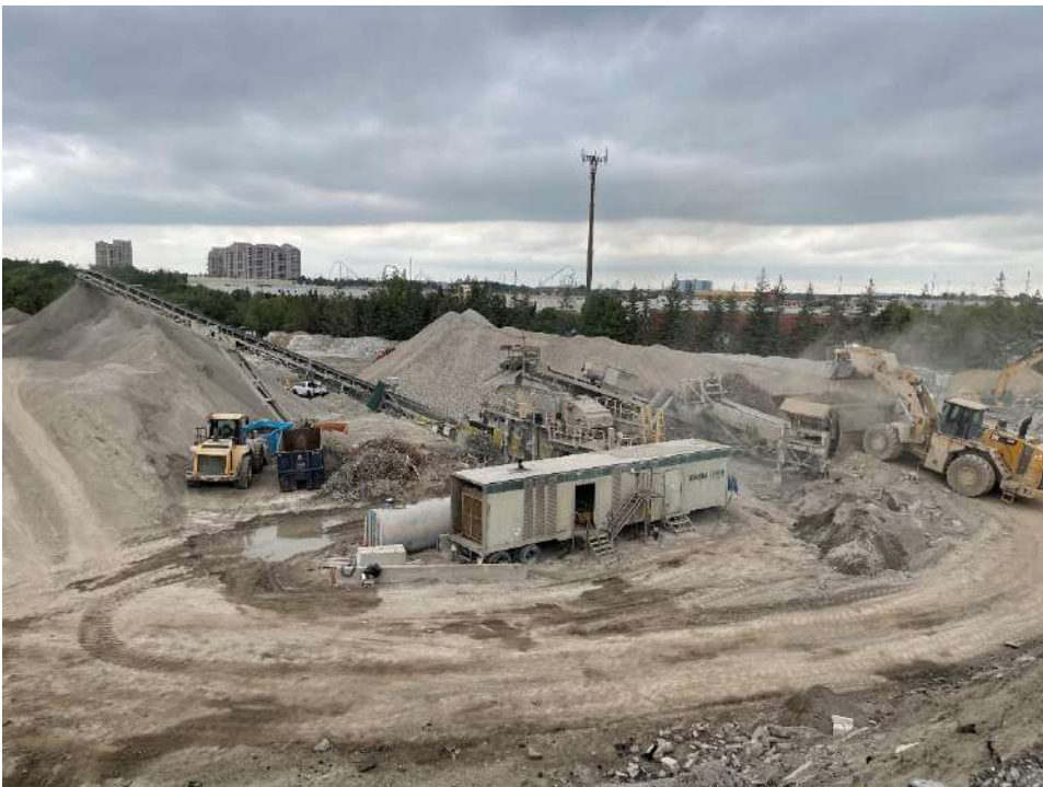
Photo (4): Strada Crusher at 1667 Creditstone Rd, Concord, ON – Producing RCA
