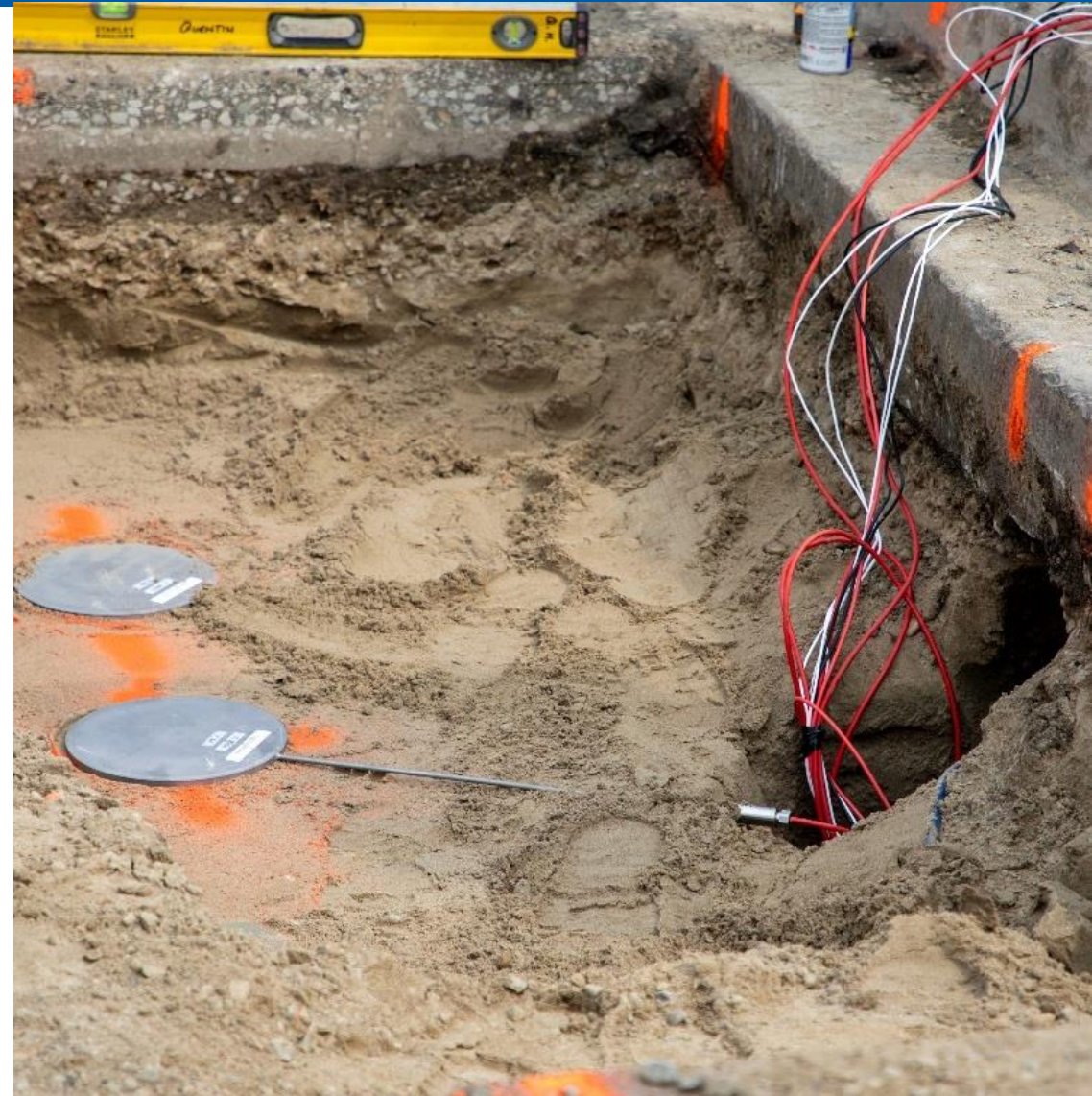
Installation of sensors for high RAP trial Leslie Street, City of Richmond Hill
